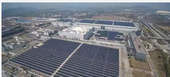
Wuhan Huaxing rooftop-distributed photovoltaic power generation project
