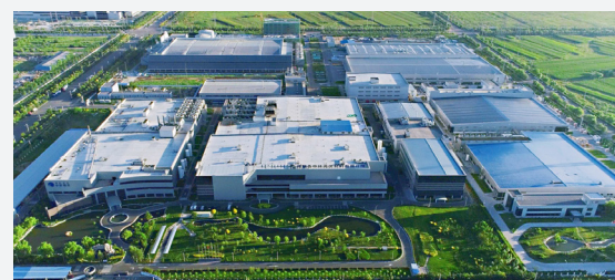
Aerial view of Inner Mongolia-Zhonghuan Industry City
