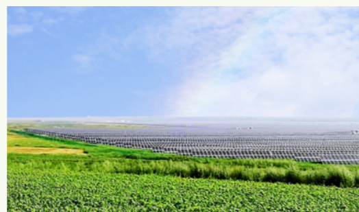
Anmeng Photovoltaic Station in Inner Mongolia
