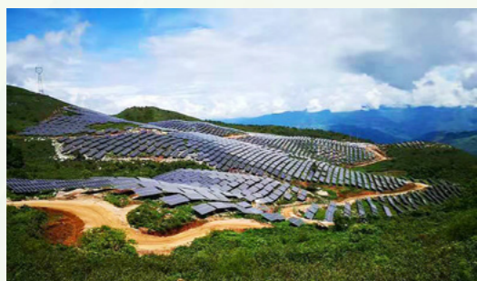
Lincang Photovoltaic Station
